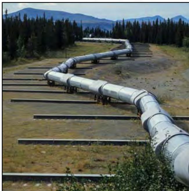
Fig. 8. The Trans-Alaska Oil Pipeline resting on concrete beams which can allow lateral ground movement where it crosses the active Denali Fault.
